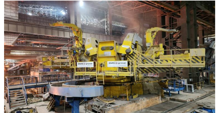
Ladle Turret at SMS-2 in BPSL
